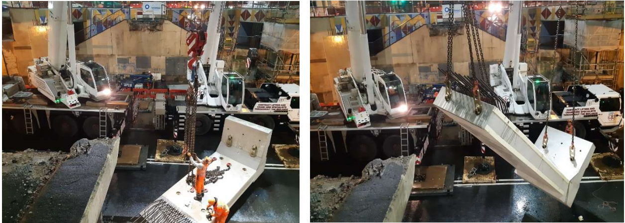
Figure 8 – Installation of OSM abutment panels, preparation [Photo courtesy of Tarmac]
